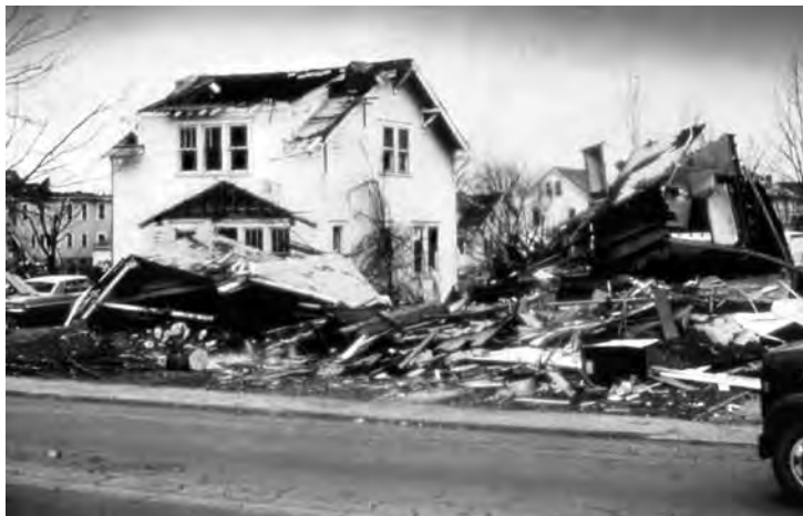
Badly damaged houses due to high winds in Kansas.
