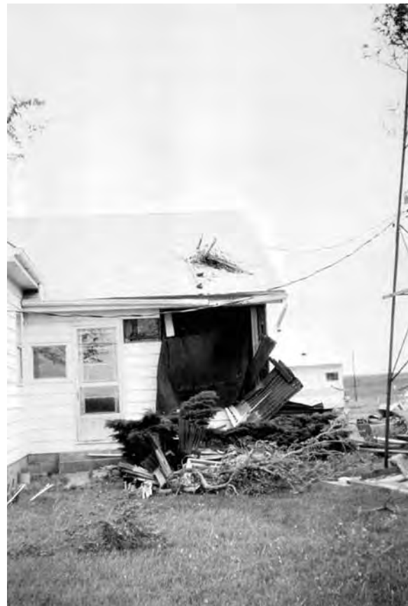
House damaged by fallen trees in Nebraska.
