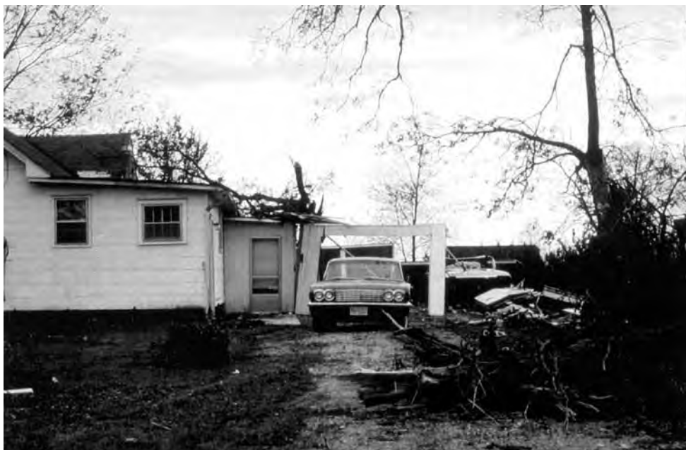
House damaged by fallen branches due to a passing windstorm.
