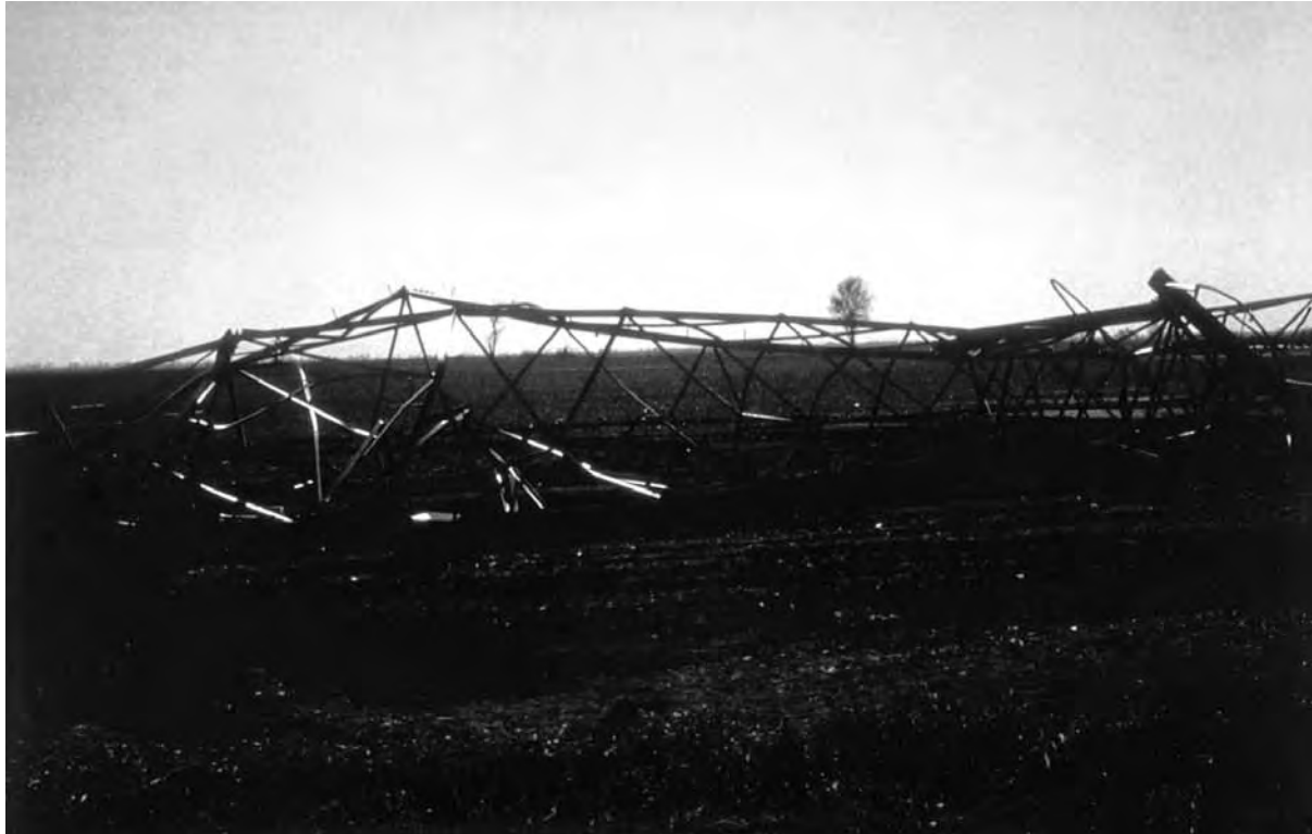
A fallen power pole, downed by high winds in Illinois.
