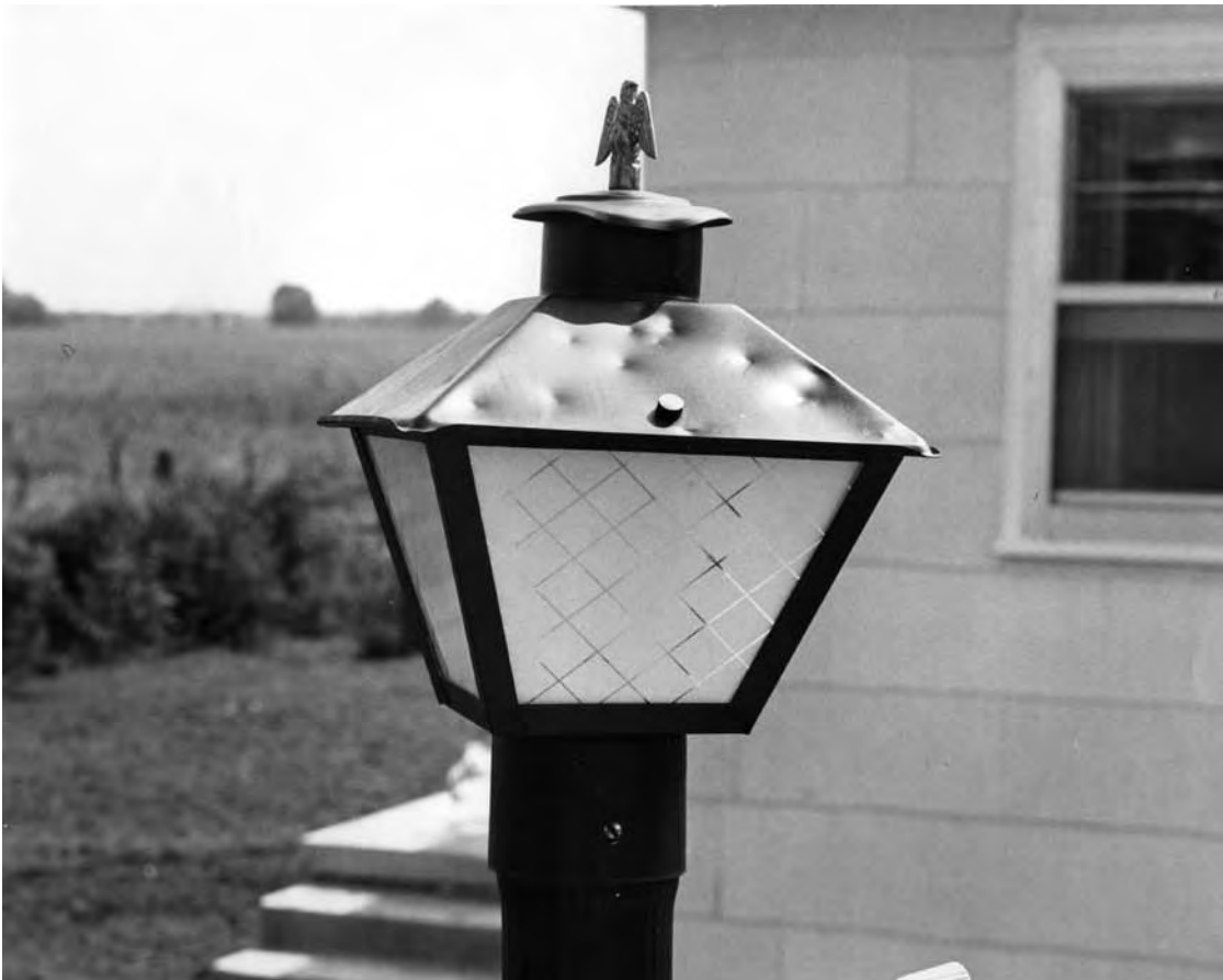
Hailstone dents in the metal cover of an outside light at a farm home in Kansas.
