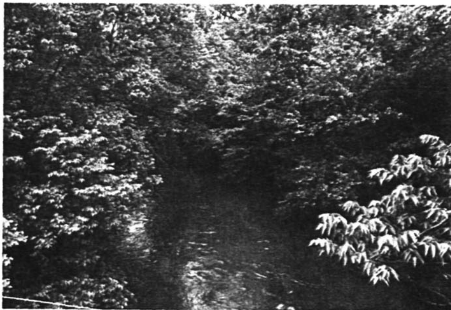
Figure 16. Main ditch of Saline Branch Drainage District, 1974, with 40 years' growth of trees, badly in need of clearing.
