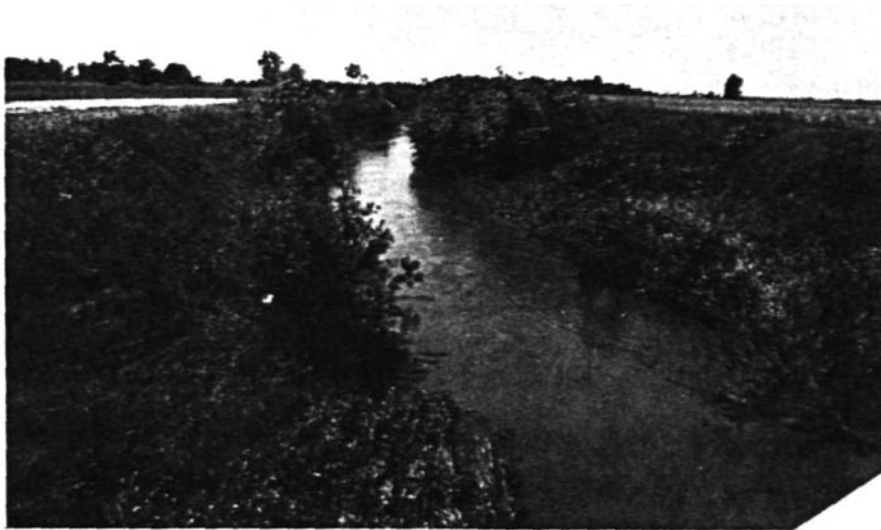
Figure 15, Main ditch of Beaver Lake Drainage Ditch in 1974, a well-maintained channel but in need of some brush removal.
