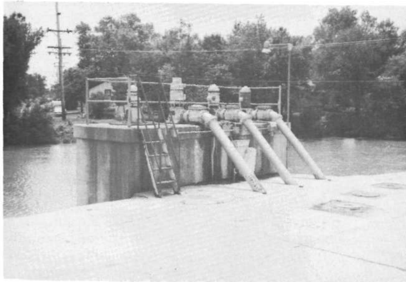
Figure 6. Intake structure of water treatment plant
