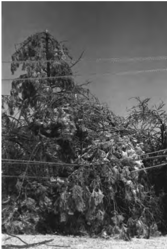
Trees and wires bent down by heavy snow and ice loads, as seen in central Illinois on December 18, 2008.
