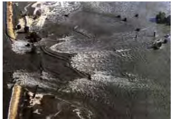
Figure 16. A levee breach that occurred near Quincy, Illinois, on June 19.
