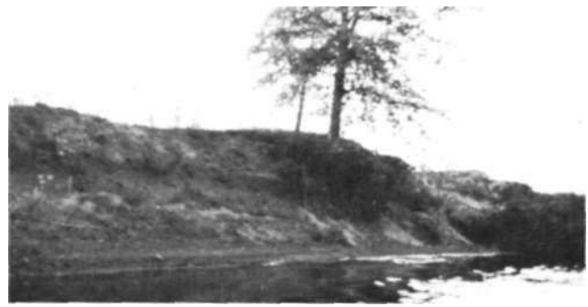
FIGURE 11 Also in Indiana some locations along the Kankakee River are bare of vegetation. Bank erosion is evident at these locations.
