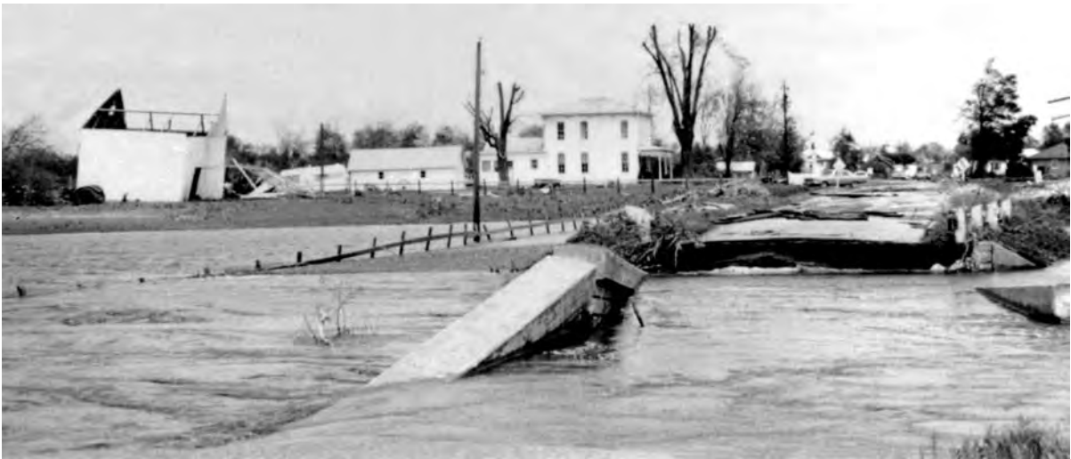
Flooding near Pontiac has washed out a bridge, as seen on January 9.
