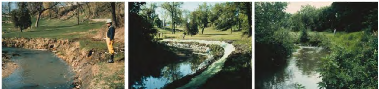
Figure 8. Stream restoration at station N2 shows pre-restoration conditions in 1991 (photo on left), mid-restoration in 1992 (middle photo), and post-restoration in 1993 (photo on right)
