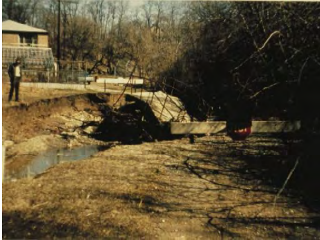
Figure 4. Damaged infrastructure on the South Branch from "flashy" storm events during 1990 in Washington Park
