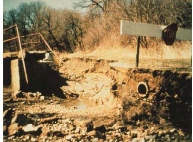
Figure 5. View upstream at the South Branch erosion site at Washington Park in 1990
