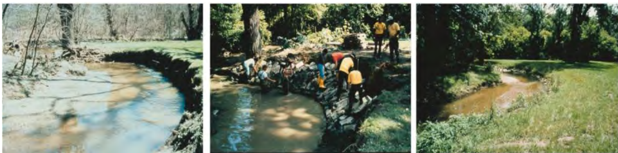
Figure 9. Stream restoration applied at station N1 before restoration in 1991 (photo on left) during construction in 1992, and post-restoration in 1993
