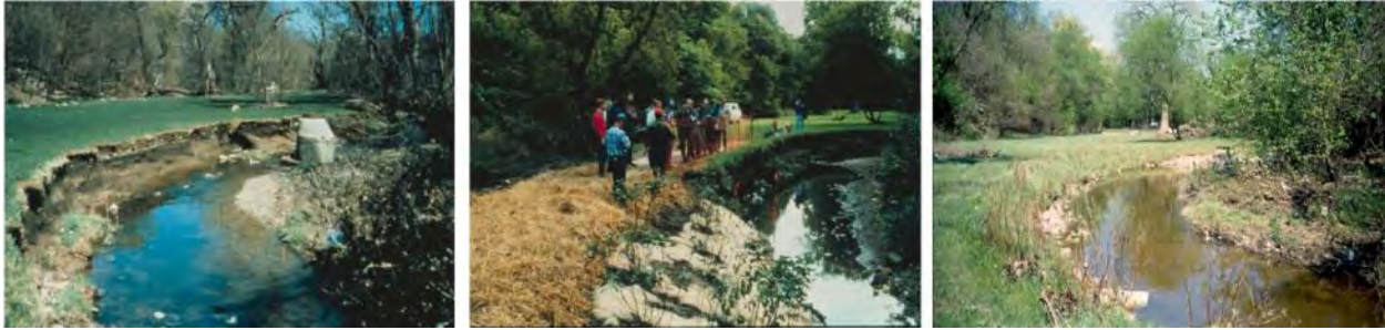
Figure 11. Stream restoration at station S1 shows pre-restoration conditions before 1991 (photo on left), mid-restoration conditions in 1994 (middle photo), and post-restoration conditions in 1995 (photo on the right)
