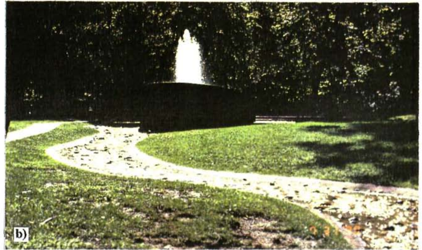
Discharge fountain and channels conveying ground water to the lake
