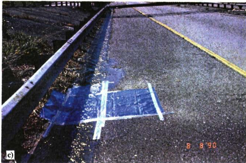
Covered road drain/
