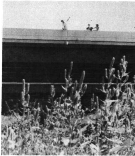
Figure 13. Sampling station 1, bridge on new U.S. Highway 51
