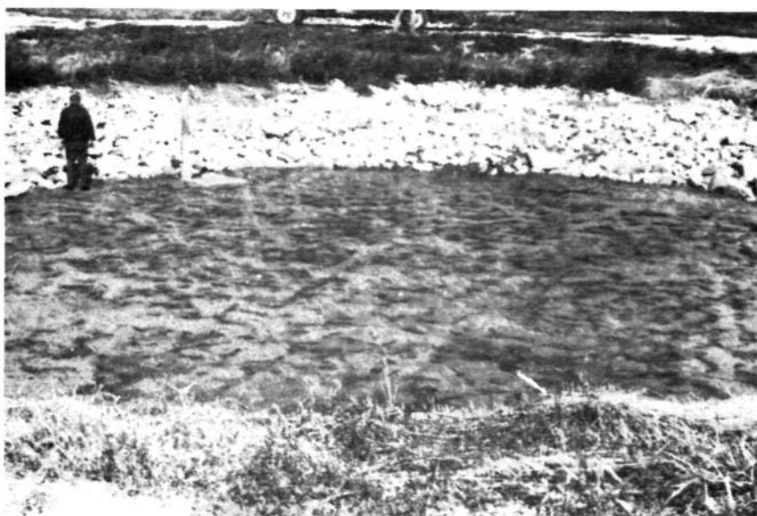
Figure 14. Lagoon bottom sand filter at Liberty
