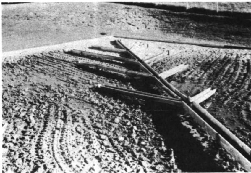
Figure 19. Distribution system for intermittent sand filter
