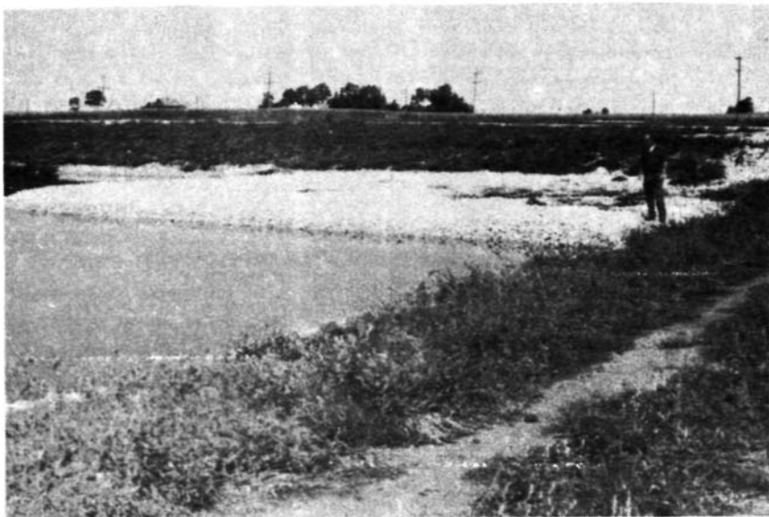
Figure 26. Submerged rock filter at Paw Paw
