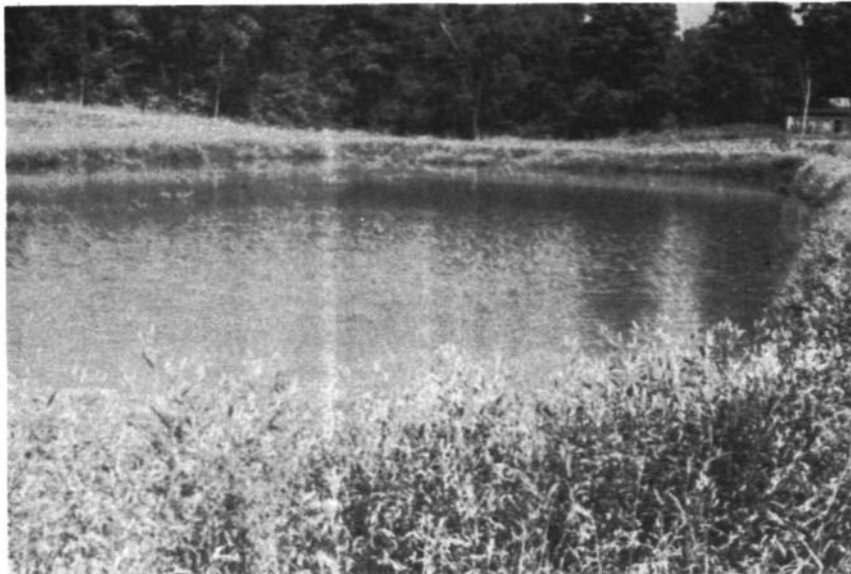
Figure 15. Lagoon bottom sand filter at Teutopolis
