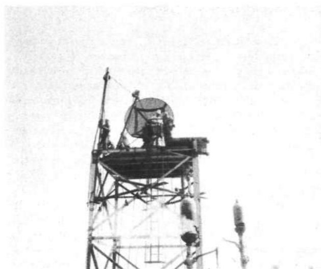
FIG. 159. —RADAR TOWER DURING CONSTRUCTION.
