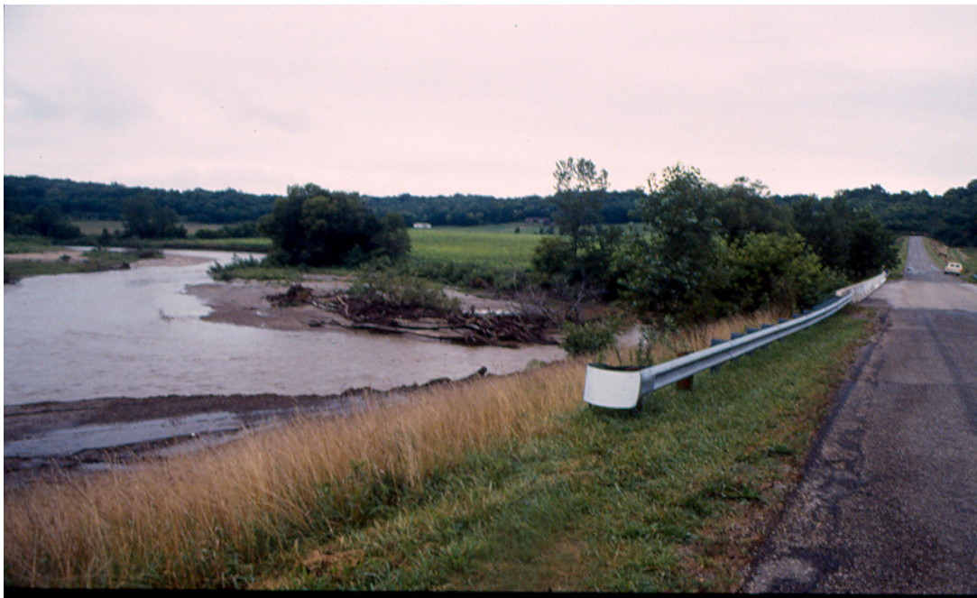
Photo 3. Picture of Benedict Bridge
