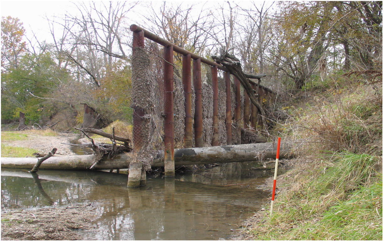
Photo 1. Exposed active gas pipeline with pipe protection along lower Senachwine Creek (Pipelines are data for interpretation of channel incision or migration)
