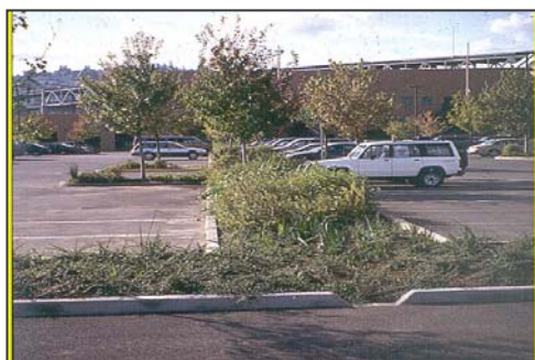
Bioretention in parking lot Photo courtesy of NRCS
