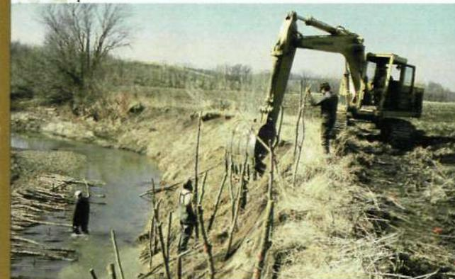
Willow posts are driven into holes made by an excavator with a metal ram.
