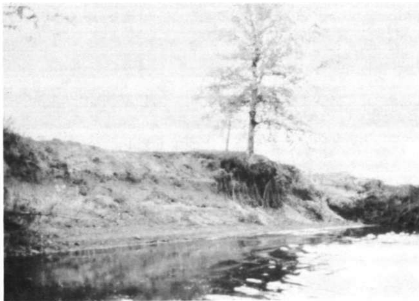
b. Bank erosion
