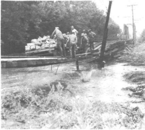
FIG. 2. AN 80 FOOT WASHOUT ON THE ILLINOIS TERMINAL RAILROAD NEAR ITS MACKINAW RIVER BRIDGE WEST OF MACKINAW.
