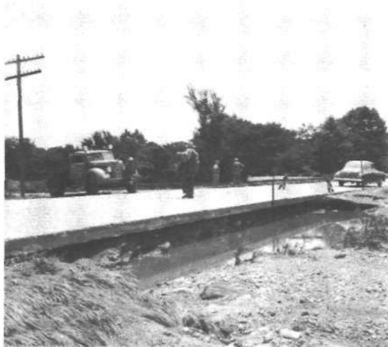
FIG. 4. AN UNDERCUT SLAB ON ROUTE 150 WEST OF MACKINAW DELLS BRIDGE.
