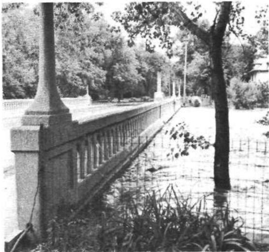
FIG. 26. VERMILION STREET BRIDGE, (looking south), AT PONTIAC, ON 11 JULY 1951; ABOUT 0.5 FOOT BELOW CREST.
