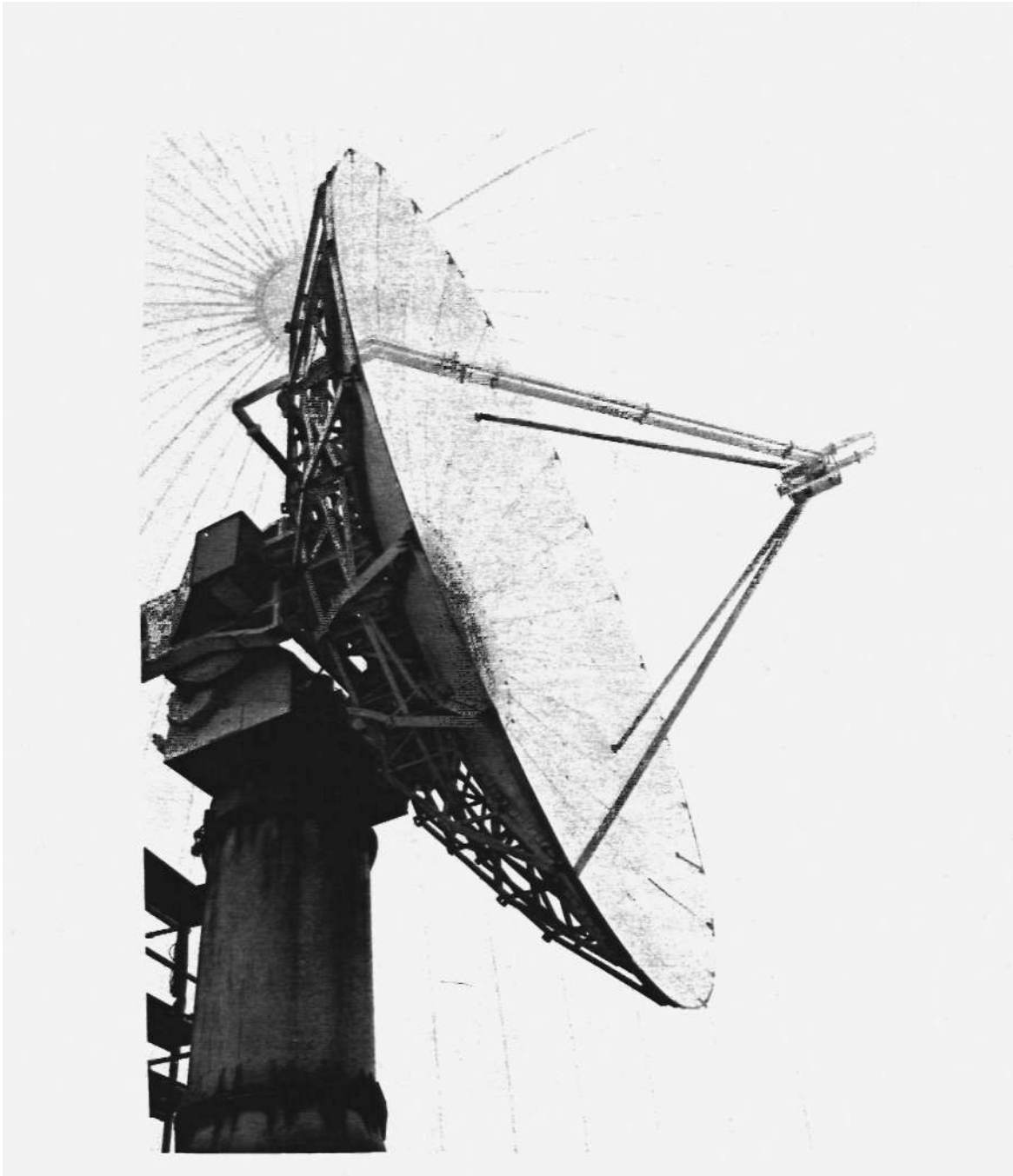
The antenna of the CHILL radar inside its radome. The design, construction, testing, and operation of this unique weather radar was one of the major technological achievements of the Atmospheric Sciences Group at the Illinois State Water Survey
