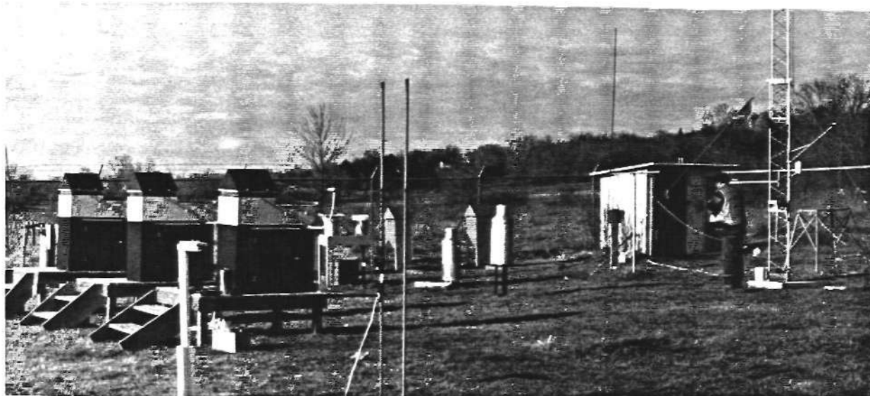
Figure 9-8. The Survey's various air chemistry samplers at Green Bay, WI site. Clyde Sweet, one of the directors of the project to sample air toxics on the Great Lakes area, is near the data shed. The three large box-like instruments on the left are wet-only precipitation collectors (for organic compounds); to their right is a wet-dry sampler; a high-volume sampler (for organic particles and vapor), a data shed, and a tower with instruments to measure winds, temperature, humidity, and solar radiation.
