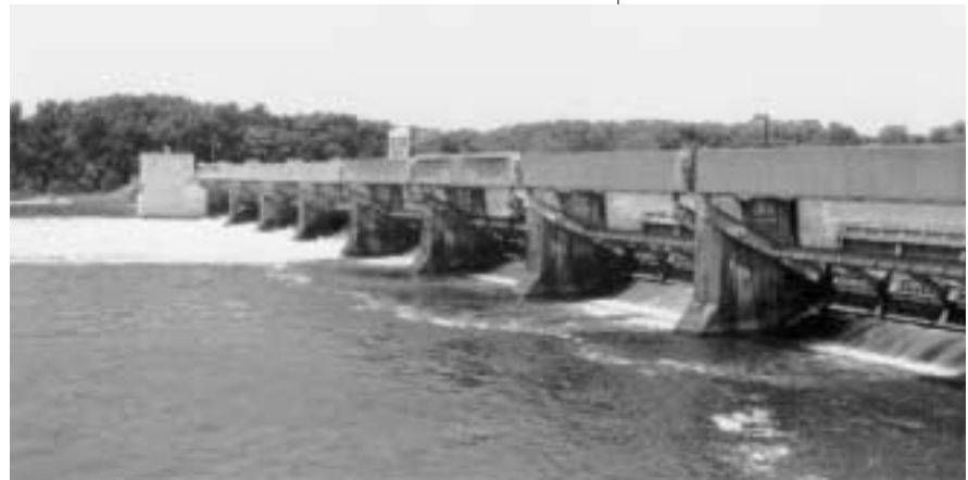
The Dresden Island Dam near Morris. Courtesy Marcia Dundore Wolter.
