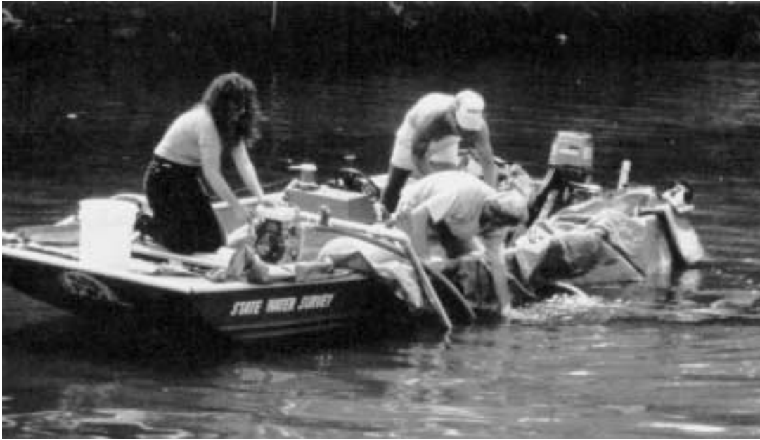
Water Survey researchers injecting a test solution into the river for a water quality study, 1990.
