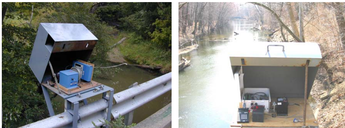
Figure 9. Streamgaging equipment: (a) Leupold & Stevens data logger and (b) CR10X data logger
