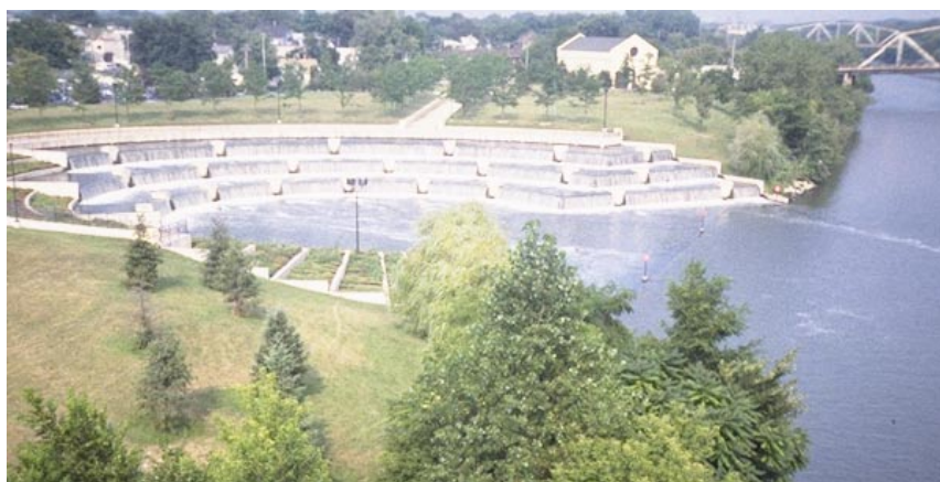
Figure 4. SEPA Station 3 outfall
