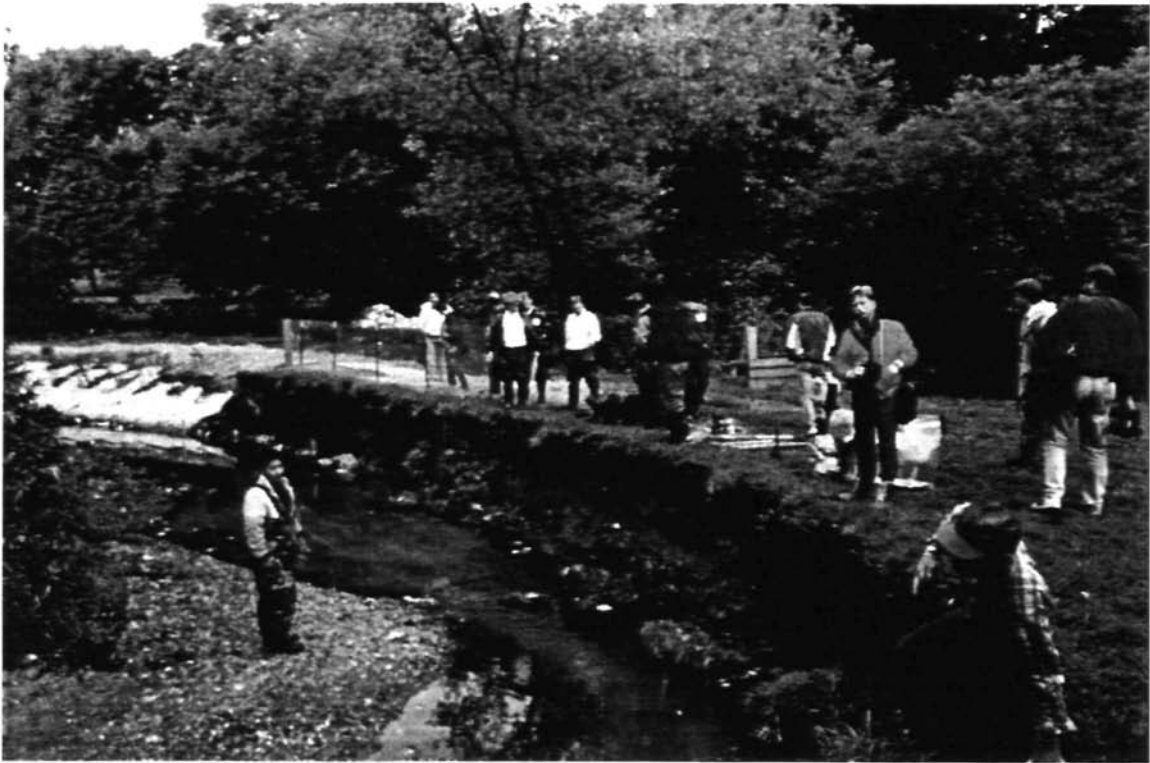
Figure 8. Workshop participants check out site in various stages of installation.
