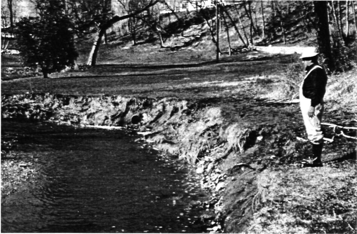
Figure 2. A major erosion site in Powell Park
