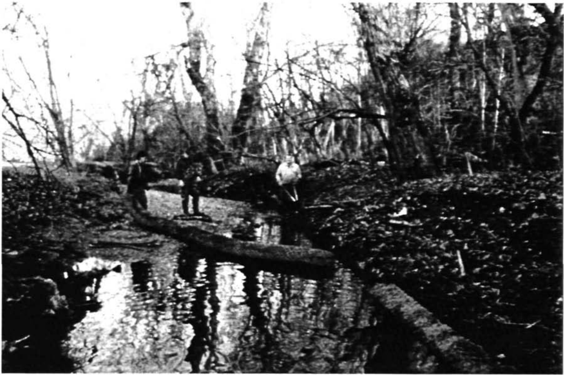
Figure 7. Fiber rolls installed at toe of streambank.
