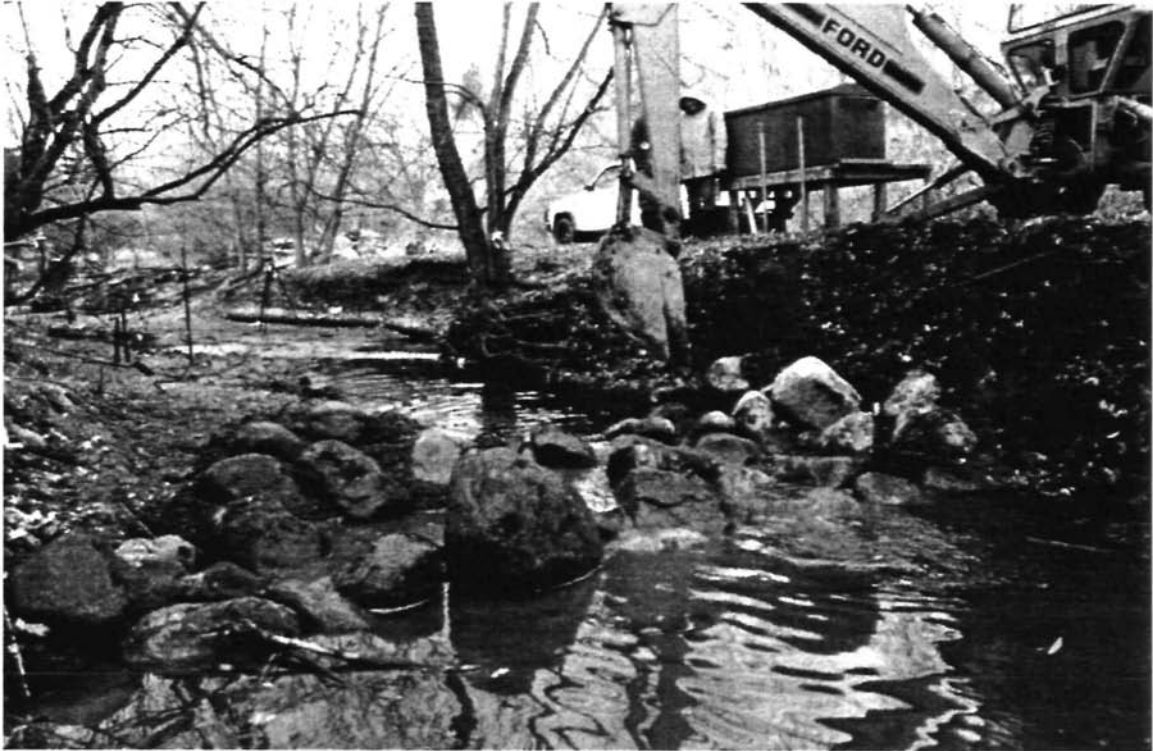
Figure 11. A tractor moves the large boulders of one of the stone weirs in Washington Park.
