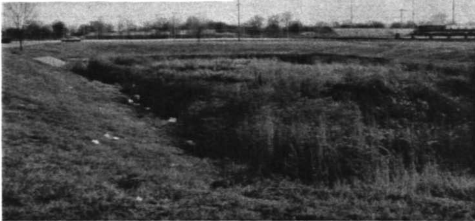
Storm detention basin for Bistate Development Agency station garage
