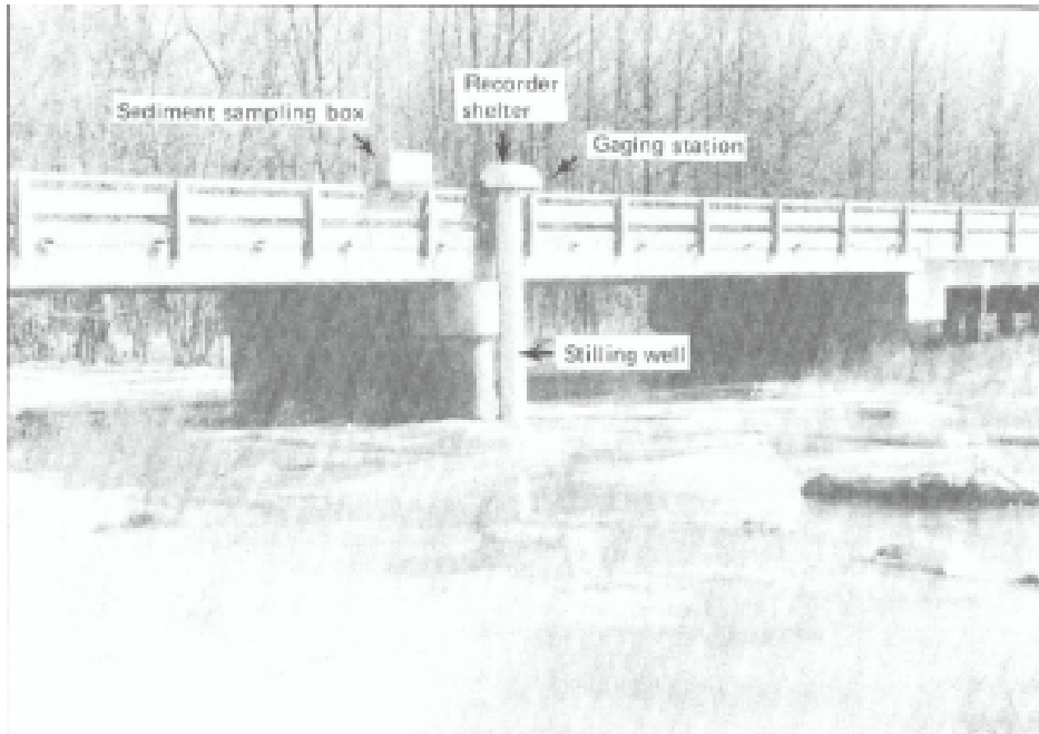
Figure 42. Gaging station installation at Route 146
