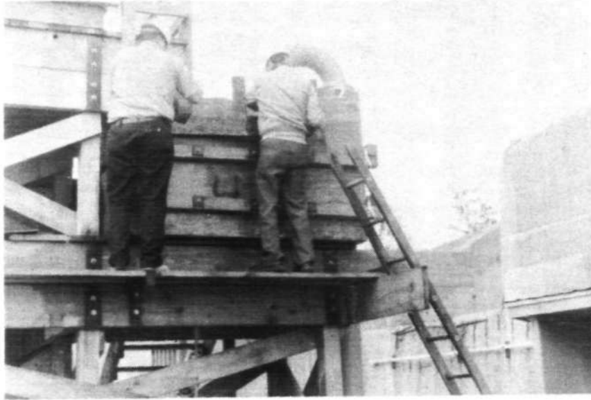
Figure 16. Clamping partitioned weir plate in place on 10-foot free-fall weir
