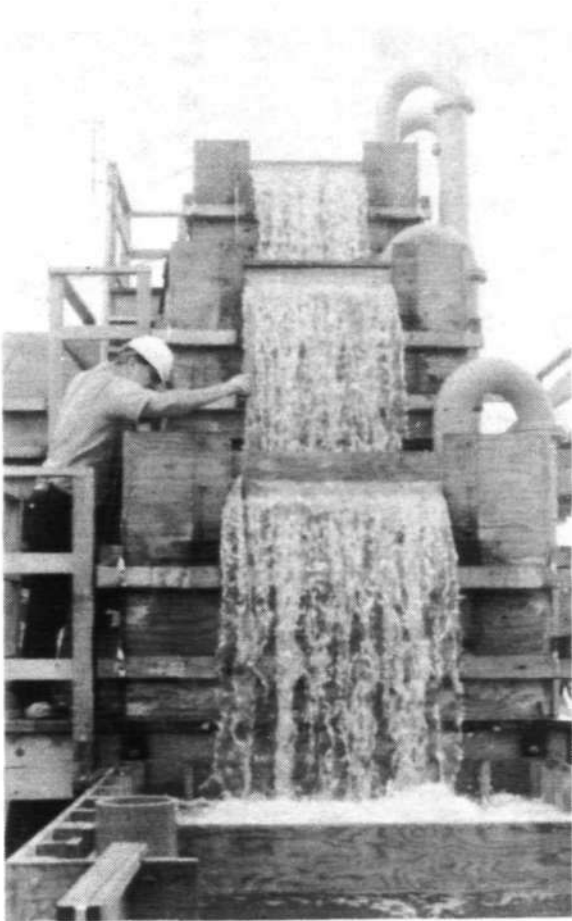
Front view of 15-foot step-weir
