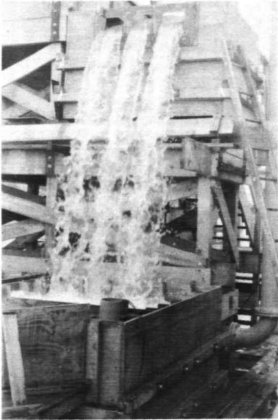
Front view of three-partition, 10-foot free-fall weir at high flow
