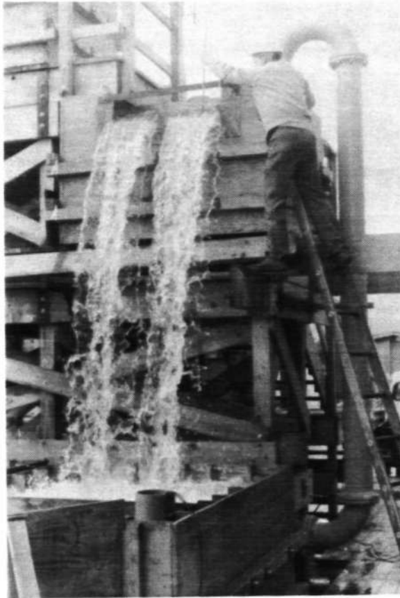
Front view of two-partition, 10-foot free-fall weir at high flow
