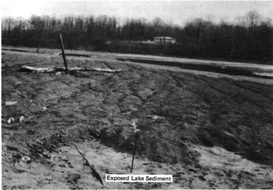
Figure 4. Lake sediment remaining on the old lake bottom after spillway failure
