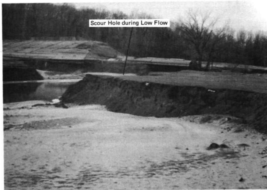
Figure 12. Scour hole just upstream of Lake Charleston spillway after its failure
