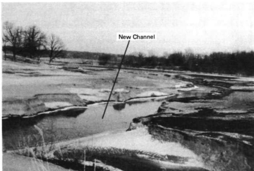
Figure 13. New stream channel which developed after the spillway failure at Lake Charleston
