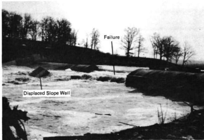
SPILLWAY AFTER FAILURE
