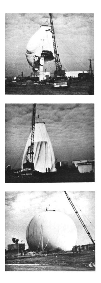
Figure 1. Sequence of photographs showing the erection of the radome over the 10am antenna in Illinois
