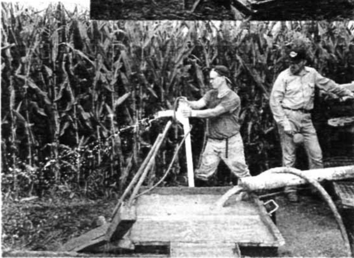
(top) Installation of a 2-inch observation well. (left) Development of an observation well. (right) Set-up of southwest aquifer test. Test well is in the background.
