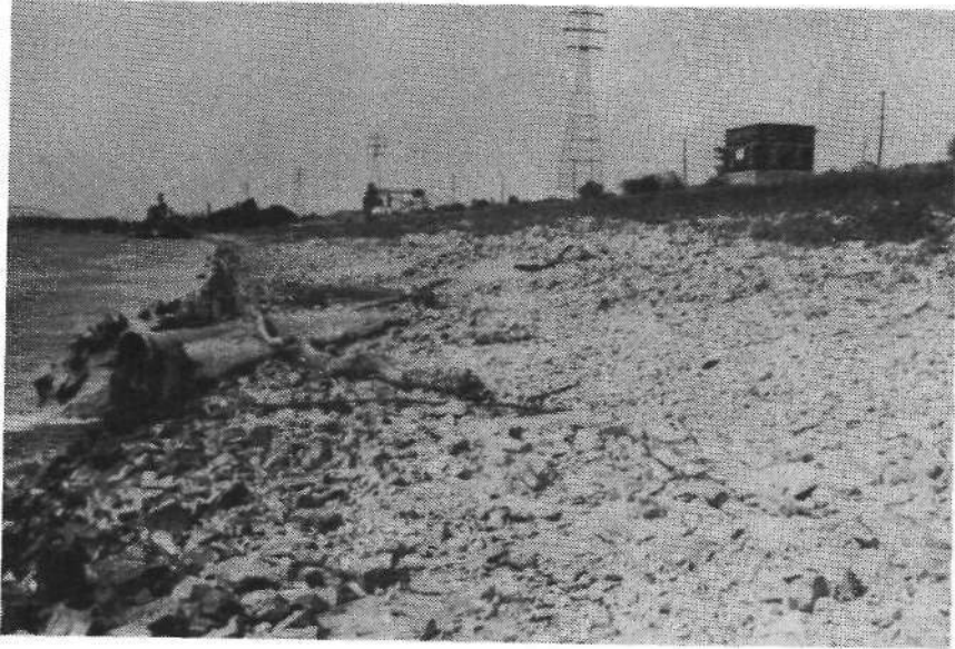
Figure 10. Outlet of stockyard gravity line
