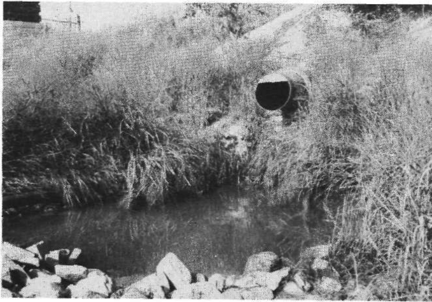
Figure 11. Outlet of Hi-line
