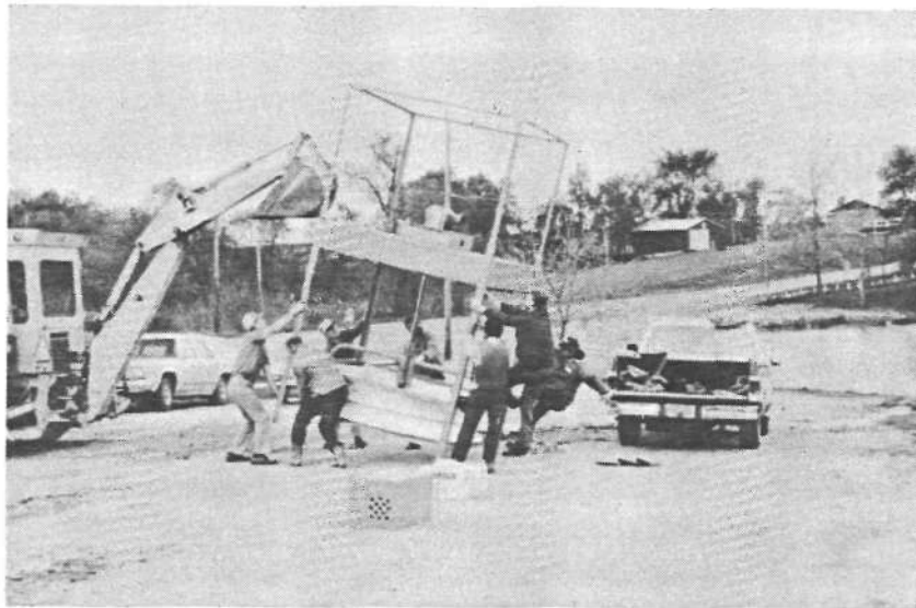
Figure 1. Completely assembled aerator prior to its installation
