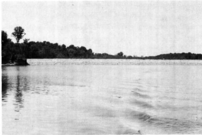
Figure 1. Main dam on Cedar Lake
