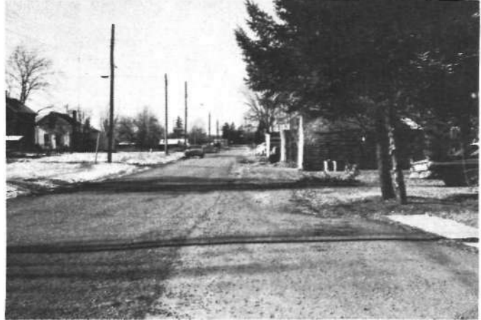
Figure 13. Flat terrain and indeterminate drainage pattern typical of much of the upstream basin of Sewer District No. 8
