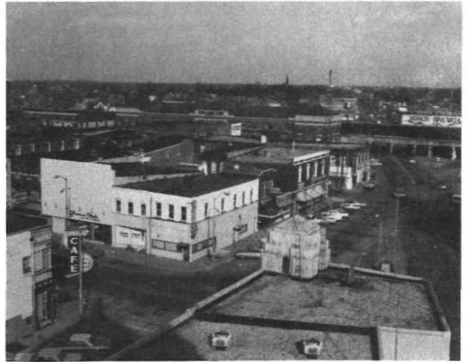
Figure 69. Street scene in the commercial area of Boneyard Creek basin
