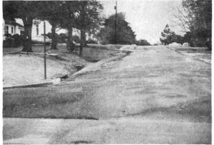
Figure 19. Ditch along street in Crane Creek basin
