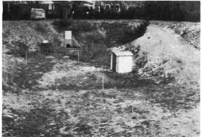
Figure 10. Outlet of the single storm drain in the Woodoak Drive basin
