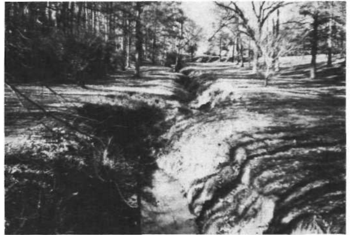
Figure 28. Open channel which is representative of most of the drainage in Third Fork basin
