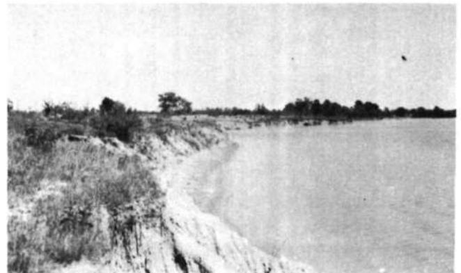
FIG. 14. BANK EROSION NEAR STATION R52
