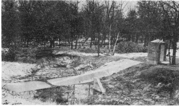
Fig. 25 - U.S.G.S. gaging station at West Frankfort Reservoir; artificial concrete control and concrete water-stage recorder shelter.
