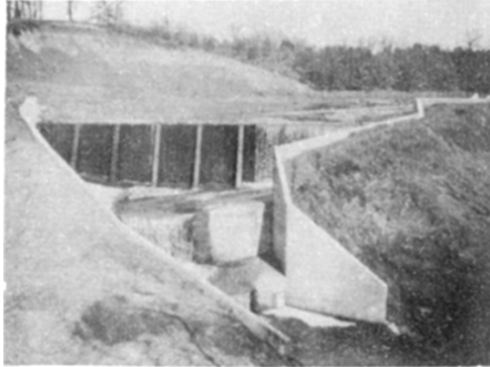
Fig. 13 - Concrete steps in spillway channel below spillway crest at Lake Bracken. Photograph taken prior to installation of gaging station.
