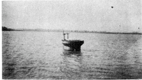
Fig. 18 - Intake tower with staff gage in Carbondale Reservoir.
