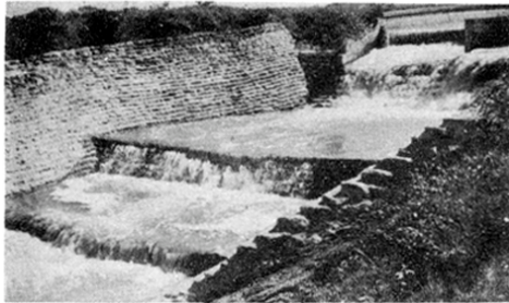
Fig. 19 - Stone steps in spillway channel below spillway crest at Carbondale Reservoir.
