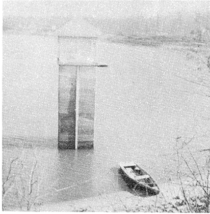
Fig. 21 - Staff gage mounted on concrete intake tower in Centralia Reservoir.
