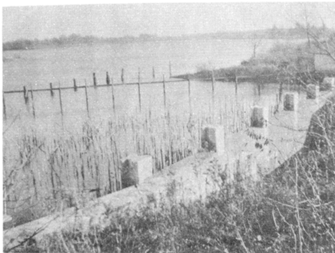
Fig. 26 - Spillway crest at West Frankfort Reservoir.
