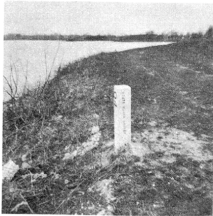
Fig. 17 - Silt range marker located on dam at Carbondale Reservoir
