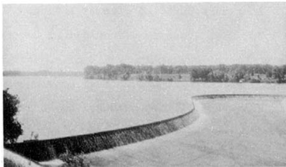
Fig. 10 - Concrete Spillway at Lake Bloomington.
