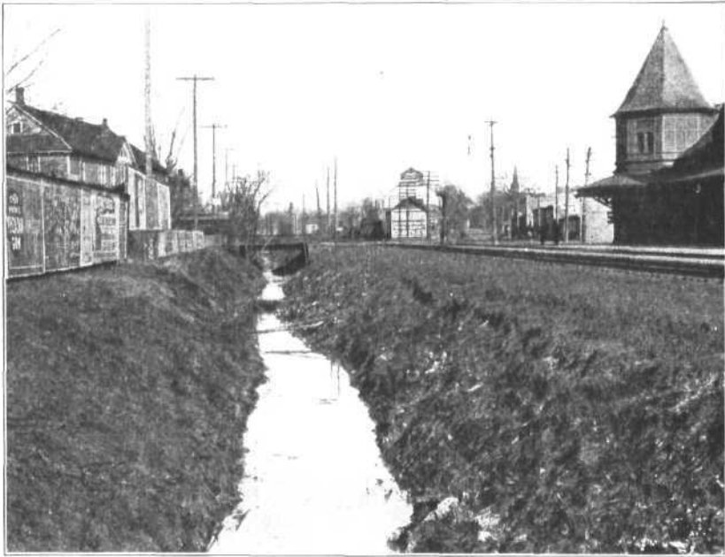
Figure 23.—Cedar Creek opposite station of Santa Fe Railway, Galesburg.
