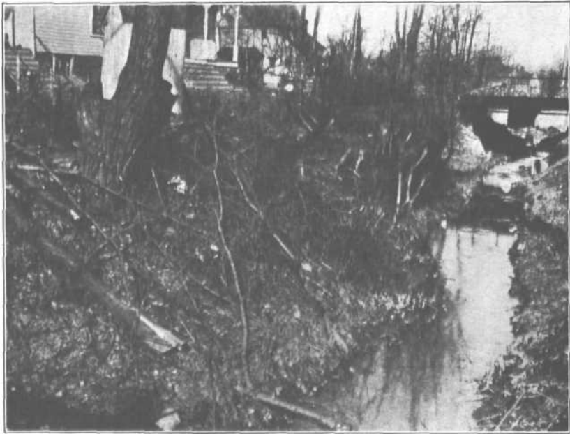
Figure 21.—Cedar Creek at Kellogg Street, Galesburg, showing large sewer entering creek within 40 feet of house.
