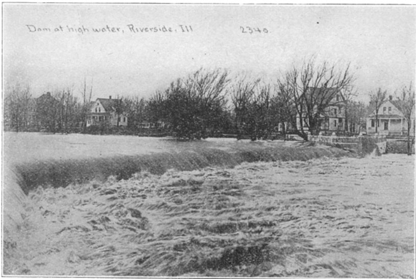
Dam at High Water, Riverside, Ill.
