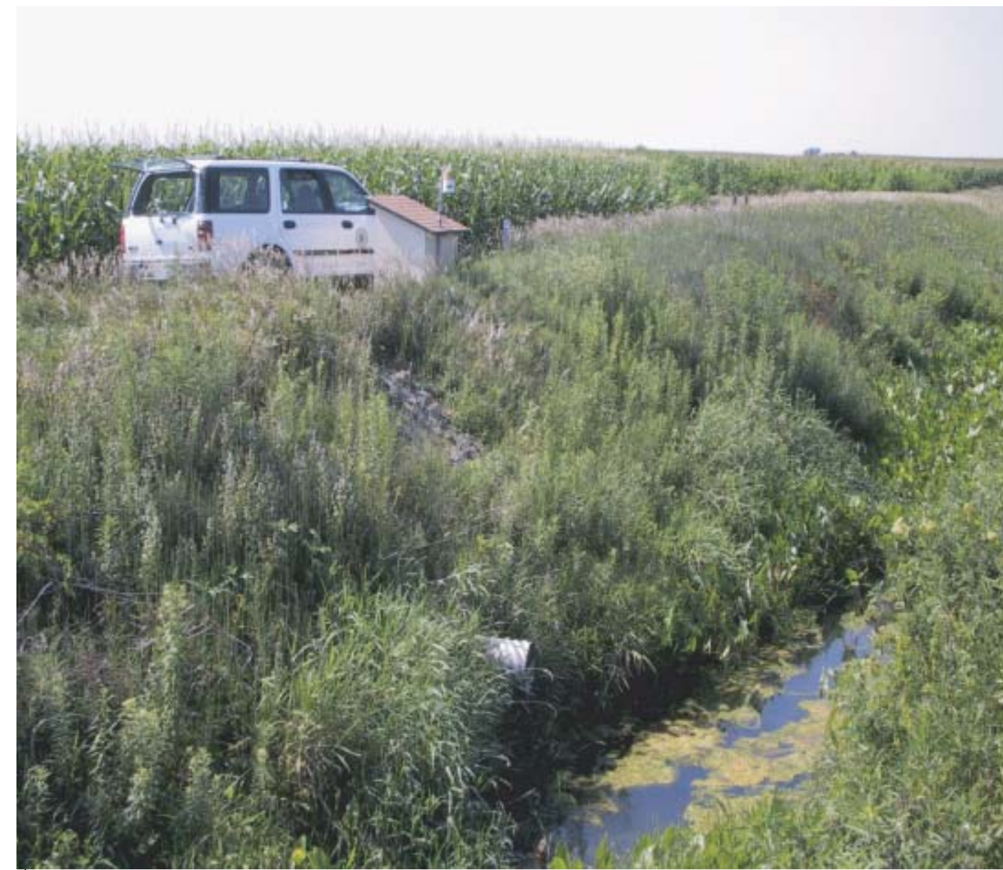
Big Ditch at Site 9. A tile drain is shown in the lower-middle part of the picture. The picture was taken in mid-summer when there was little drainage from the tiles.
